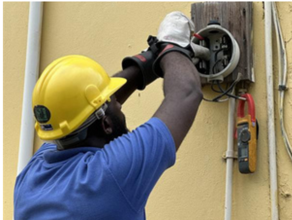
Joash Marquis replacing a meter
