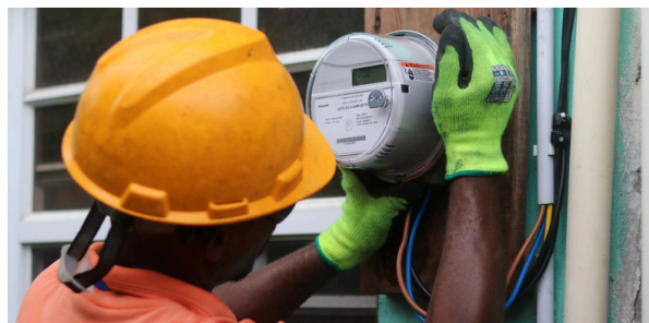
LUCELEC Contractors Kings Electrical on site of a meter replacement
